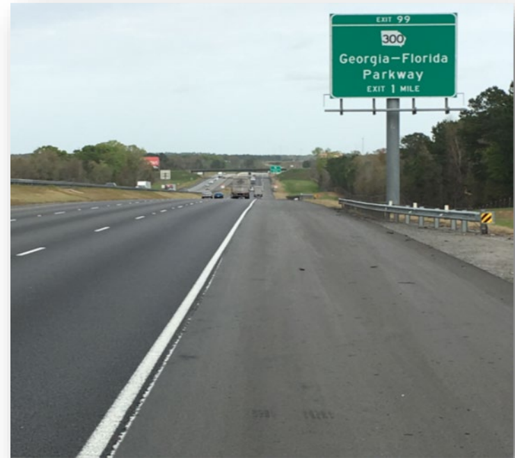
Exit 99 - Crisp County
